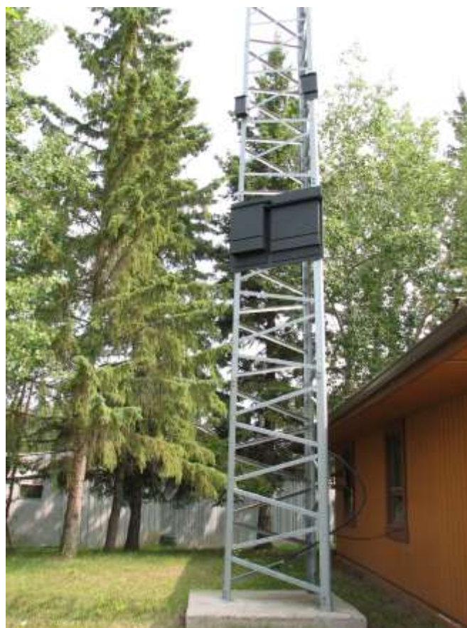
Figures 1 – 5. Erecting four bat houses at Waskehegan, July 2018.
